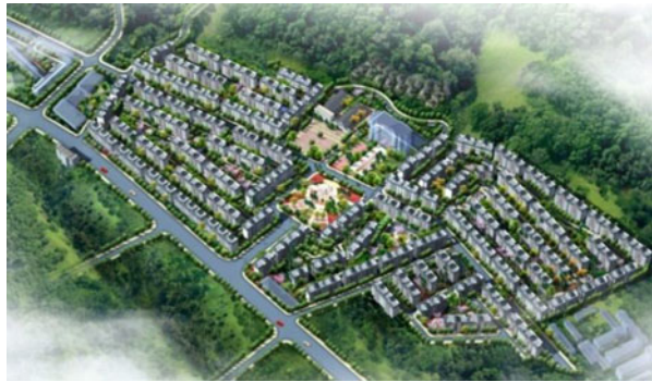
Fig. 14.8 Complex of dwelling buildings in South-Western P.R. China, formed by 94 4- to 6-storey seismically isolated buildings (overall floor area = 280,000 m 2 ) (Eisenberg et al. 2011)
