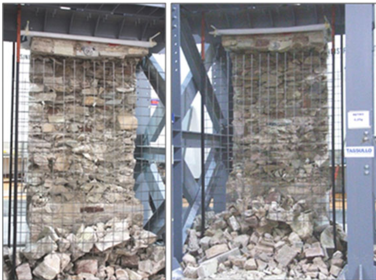
Fig. 8.19 Failure of walls 1 and 2 (Valluzzi et al. 2013)
