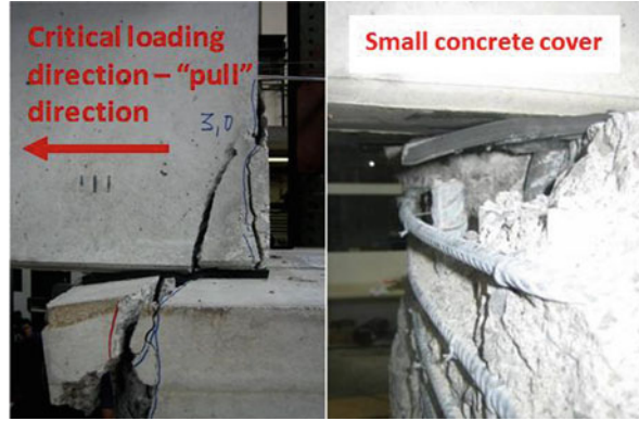
Fig. 4.34 Failure in the case of small concrete cover and in the case of the insufficient tension strength of concrete and stirrups surrounding the dowel
