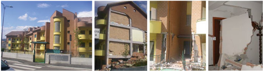
Fig. 14.22 Left : the dwelling building complex (3 buildings) of Via Borgo dei Tigli 6-8-10 in L'Aquila (Pianola area), which had been just completed before the 2009 Abruzzo earthquake. Right : damage caused to the building by this event
