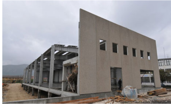
Fig. 4.7 Structural system of most precast industrial buildings designed for seismic action remained undamaged during recent Italian earthquakes
