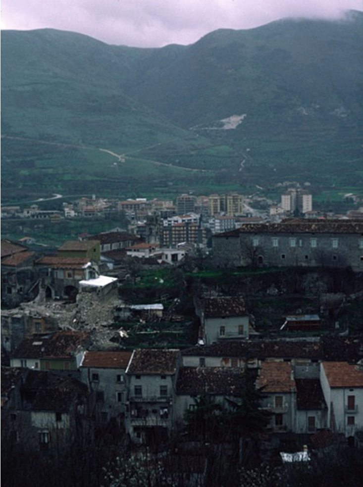
Fig. 1.6 Polla from the same location as Fig. 1.6 in 1981 after the Irpinia earthquake. Note similarity of building form and construction (Photo by author)
