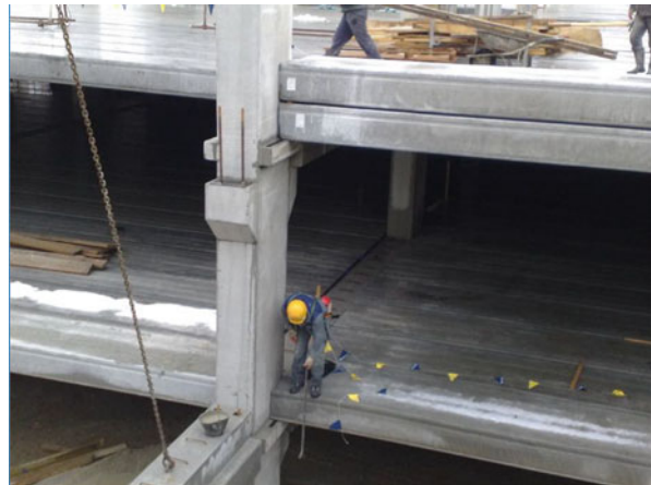
Fig. 4.5 Beam-to-column dowel connection is clearly seen in the upper floor. In the lower floor the beam has been already installed and the steel sockets will be grouted
