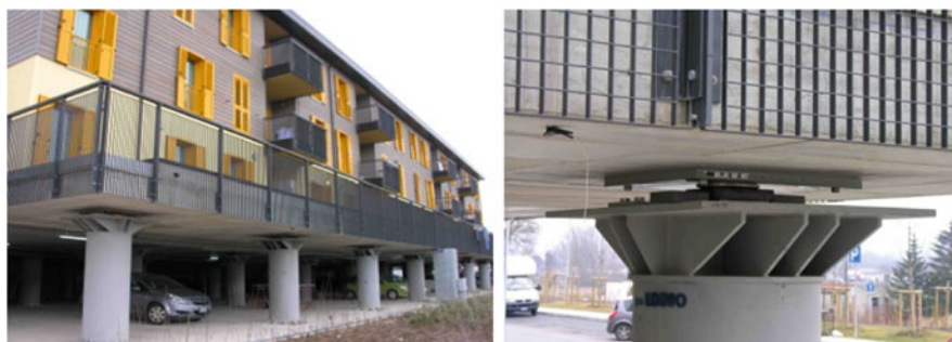
Fig. 14.20 Left: one of the 184 pre-fabricated houses (wood, or r.c., or steel structures) erected in L'Aquila to host up to 17,000 residents who remained homeless after the 2009 Abruzzo earthquake. Right: detail of one of the 40 CSS devices, manufactured in Italy, which have been installed at the top of columns (made of steel or r.c.) to isolate the supporting slabs of such houses
