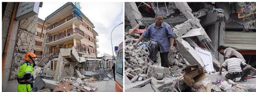
Fig. 14.26 Left: the “Student House” in L’Aquila, collapsed during the Abruzzo earthquake of April 6, 2009 ( M=6.2 ), causing the death of eight students. Right: secondary school in Dujiangyan (P.R. China), collapsed during the Wenchuan earthquake of May 12, 2008 ( M\approx 8.0 ), causing the death of 900 students
