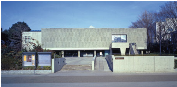
Fig. 14.4 The 4-storey National Western Art (Le Corbusier) Museum in Tokyo, retrofitted by inserting HDRBs in a sub-foundation in 1999. During the 2011 Tohoku earthquake the SI system reduced the PGA values in the two horizontal directions from 0.19 to 0.27 g at the base to 0.08 and 0.10 g at the top (Eisenberg et al. 2011)
