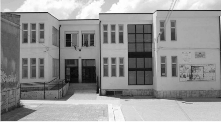
Fig. 3.10 North-east view of the building
