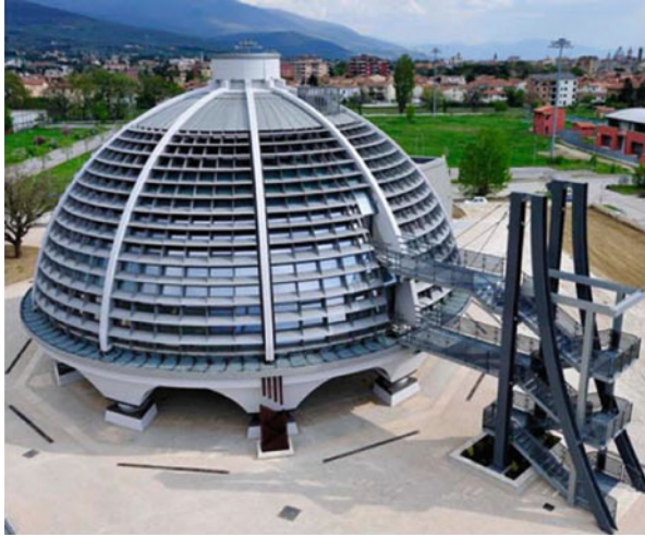
Fig. 14.17 Main building of the Civil Defence Centre of Foligno (Perugia), former seismic zone I, isolated by 10 HDRBs and certified as safe by A. Martelli in 2011
