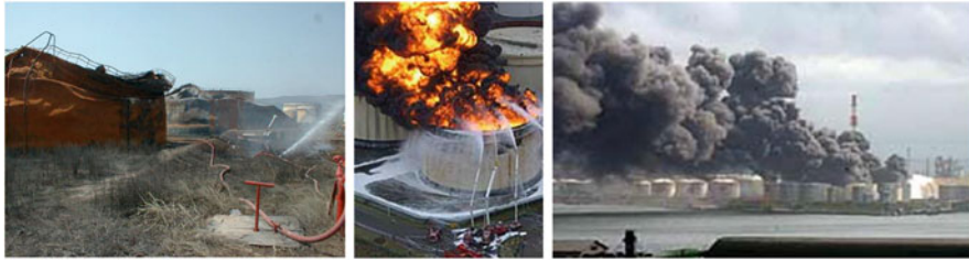
Fig. 14.27 Left : rupture of a storage tank in the Yarimca Refinery (Turkey), owned by Tupras, during the Izmit earthquake of August 17, 1999 ( M_w = 7.4 ), which caused 17,000 victims. At the centre: initial fire of one the two tanks (the first containing crude oil, the second naphtha) of the Tomakomai City petrochemical installation (Japan), caused by the two main shocks of the Off Tokachi earthquake of September 26 and 28, 2003 ( M = 8.0 and M = 7.1 ), with epicenters at 220 km from the plants. Right : propagation of the fire in the Tomakomai City petrochemical installation, during the aforesaid quake, with the consequent damage of 45 tanks (30 severely, 29 with leakage) of the 105 present
