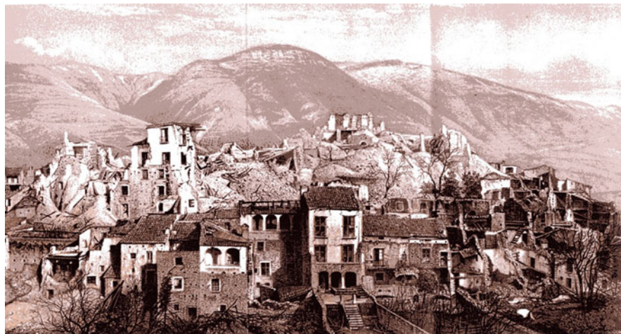
Fig. 1.5 The damage to Polla, in Irpinia, in the 1857 earthquake (from frontispiece of Mallet 1862)
