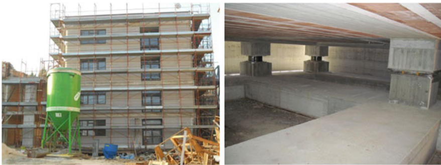
Fig. 14.18 The new block B of the Romita High School for scientific studies in Campobasso (former seismic zone 2), isolated by 12 HDRBs and 10 SDs, which was reconstructed with SI, after its demolition in 2010 (blocks A and B had been found unsafe by ENEA, CESI and the University of Basilicata in 2003 – see Fig. 14.29). The safety of the new building was certified by A. Martelli in 2013
