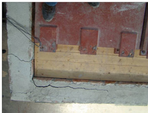
Fig. 8.7 Separation of the leaves of masonry walls during tests on the shaking table (Mouzakis et al. 2012a)
