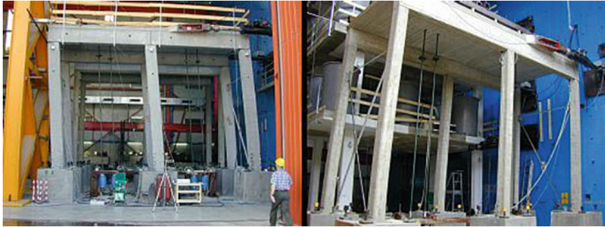
Fig. 4.17 Precast ( left ) and cast-in-situ ( right ) ECOLoader prototypes during testing
