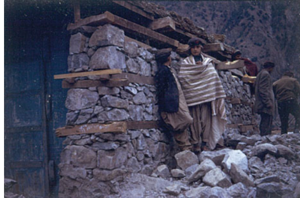
Fig. 1.8 Stone masonry buildings with roofs supported on timber columns independently of the walls, from UNESCO mission to 1974 Pattan earthquake (Ambraseys et al. 1975)
