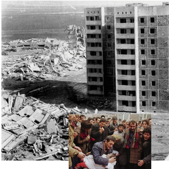
Fig. 4.2 Large panel precast structure standing among the rubble of the precast frames, which caused a terrible tragedy during the Spitak 1988 earthquake
