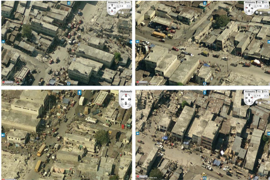
Fig. 1.19 Pictometry images of damage in the 2010 Haiti earthquake (Booth et al. 2011a)
