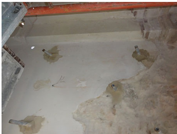
Fig. 15.6 Wall prepared for grout injection
