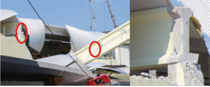
Fig. 4.11 Collapse of the beam during Emilia earthquake due to the loss of the seating; general view – left and the detail of the support – right (Bournas et al. 2013a)
