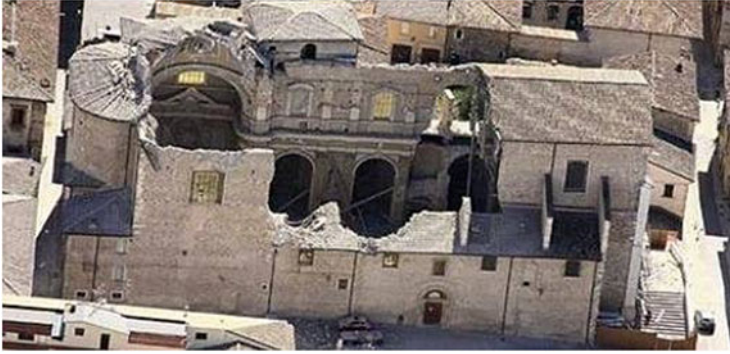
Fig. 15.4 Collapse of the roof and vaults of the church of Santa Maria Paganica, L'Aquila
