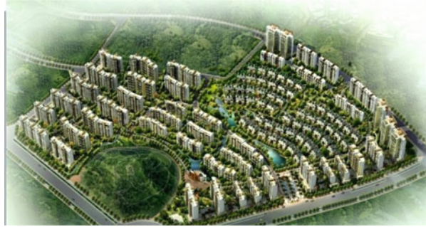
Fig. 14.7 Complex of dwelling buildings in South-Western P.R. China, formed by 82 4- to 16-storey seismically isolated buildings (overall floor area = 210,000 m 2 ) (Eisenberg et al. 2011)
