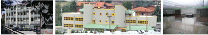
Fig. 14.29 Left : the Romita High School in Campobasso (Italy), in 2003 (when it hosted 1,300 students), before the demolition of its two most unsafe A and B blocks and reconstruction of block A with SI (see Fig. 14.18). At the centre and right : the new school of Marzabotto (Bologna, Italy, former seismic zone 3), which was seismically isolated (with the collaboration of ENEA) by means of 28 HDRBs and 14 SDs, with 500 mm diameters; it is the first seismically isolated school in Northern Italy, which was certified as safe by A. Martelli in September 2010
