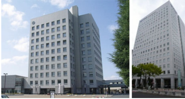
Fig. 14.3 Left : the seismically isolated 10-storey Hachinohe City Hall, near Sendai, isolated by means of LRBs. Right : the 18-storey MT Building in Sendai, isolated by means of RBs and SDs. Both buildings withstood the 2011 Tohoku earthquake undamaged (Eisenberg et al. 2011)
