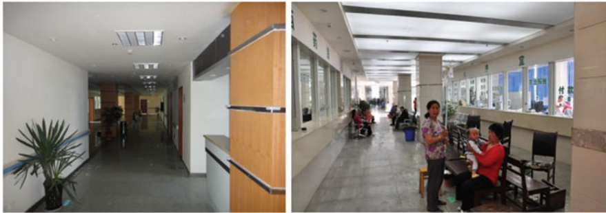
Fig. 14.11 Full integrity and operability of the isolated building of the hospital of Fig. 14.9 (Zhou et al. 2013)
