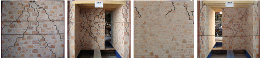
Fig. 8.26 Crack pattern of the subassembly (Vintzileou et al. 2012)
